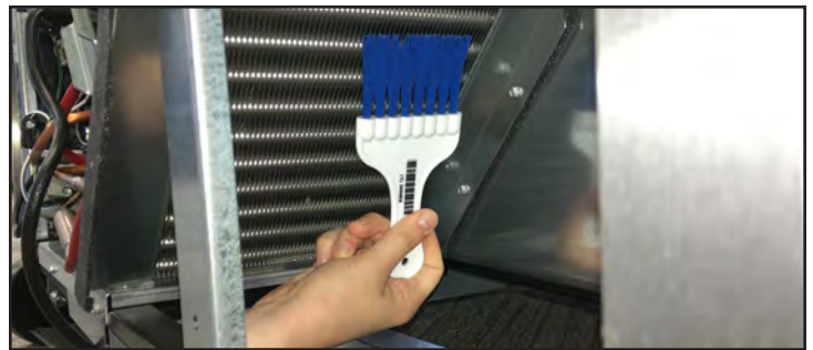
Fig. 3. Never brush across the coil fins.
