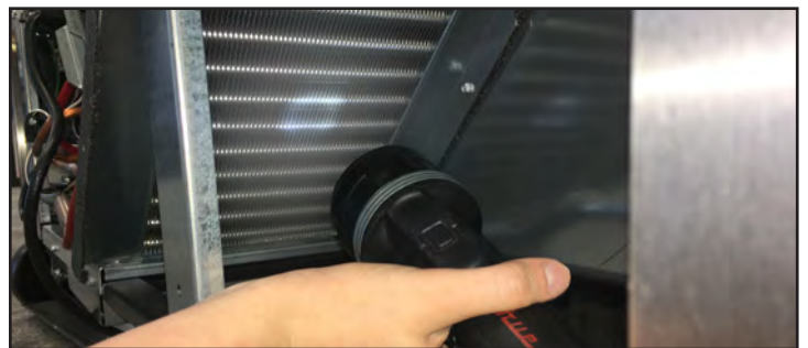
Fig. 4. Verify all blockages have been removed.
