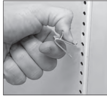
Fig. 1. Installing top tab of shelf clip.
